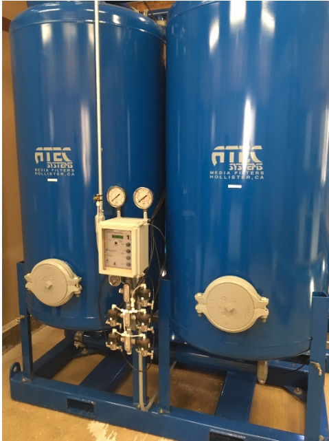
Pressure Filters Approx 8' Tall x 6' x 4'
