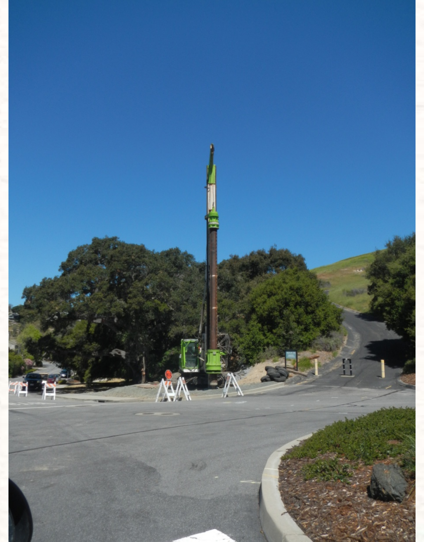
Conductor Casing Installation
